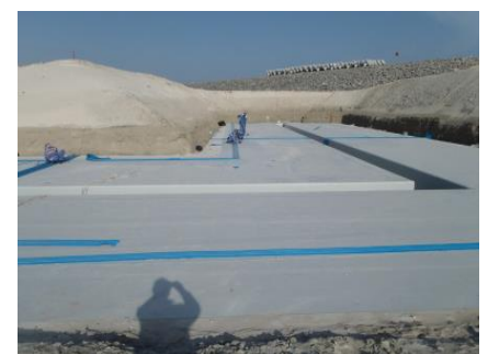
Proofex PGP & Supercast PVC applied
