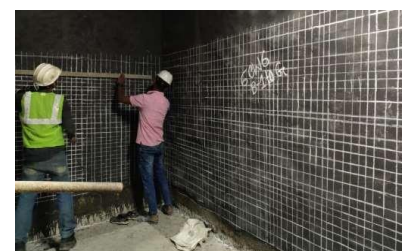
Scanning & Reinforcement position marking
